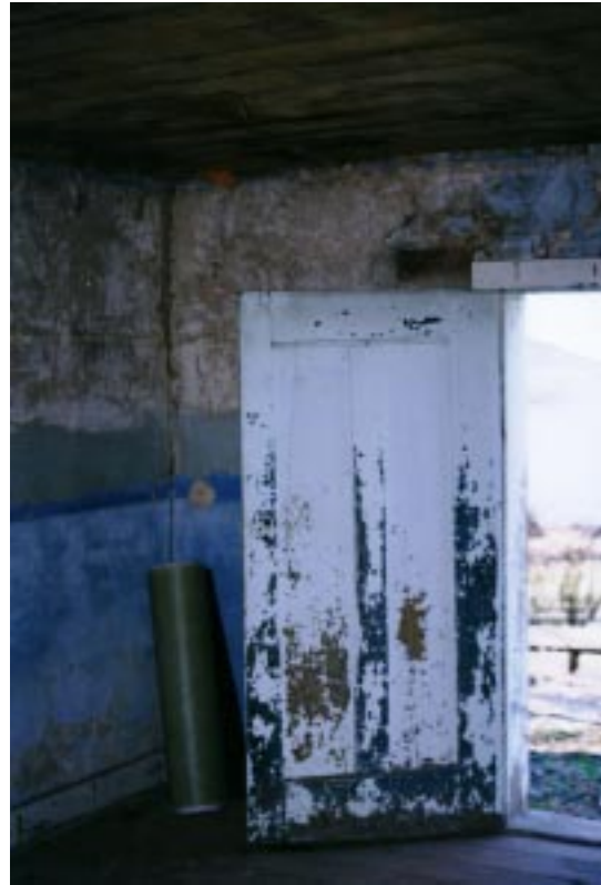
Fig. 4. This blue and tan two-panel door probably is original to the east room addition of the house.
