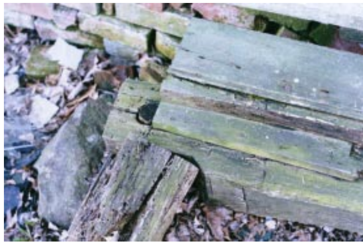
Fig. 6. The remains of the kitchen ell include these wonderfully joined pieces of the old sills.
