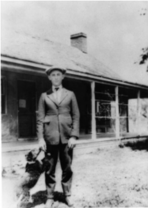
Fig. 12. As this early 20 th Century photograph shows, the Five Mile House is a link to Coles County's historic past.
