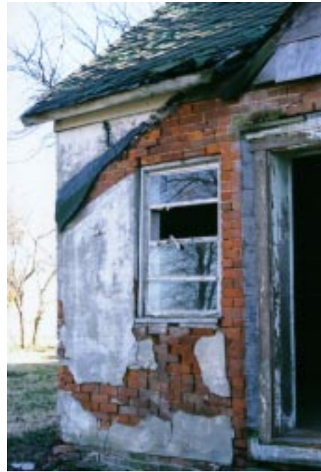
Fig. 7. The shingle paper tarred above the window on the northeast corner of the house is evidence of a kitchen ell porch.
