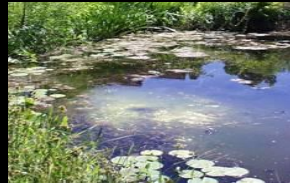
Rain garden used for natural stormwater detention
